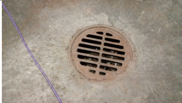
Image P23: Floor drain in mechanical space.
