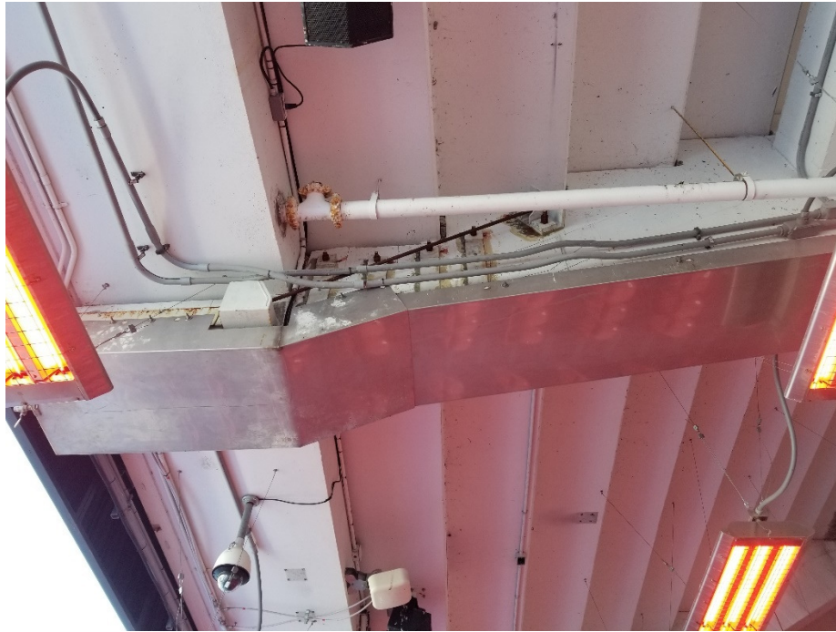
Image E22 Typical IR Heater Broken Conduit and Supports
