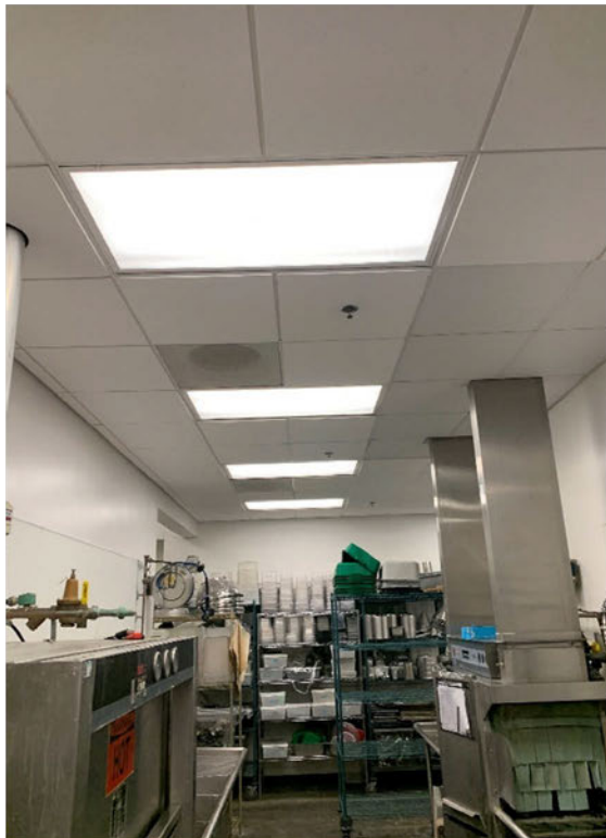
Image E44 Typical Recessed 2'x4' Lighting
