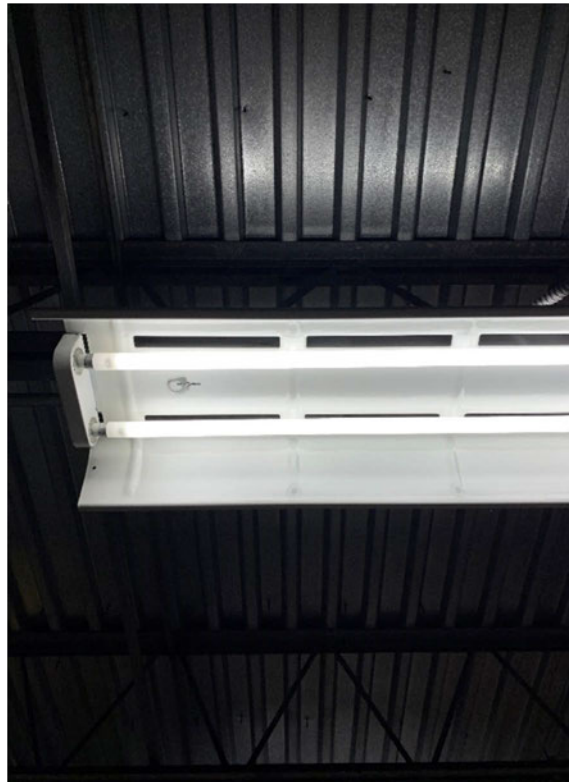
Image E52 Typical Suspended 2'x4' Fluorescent Fixture
