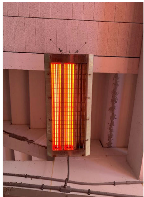
Image E21 Typical IR Heater with Element Out
