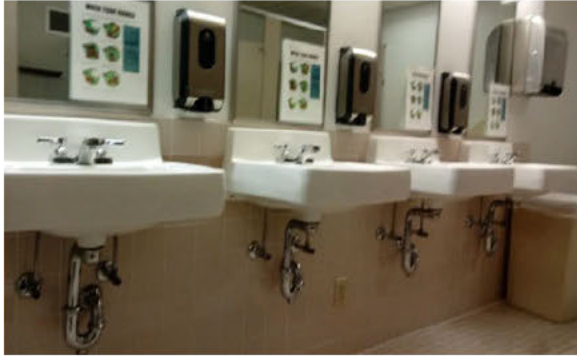
Image P9: Lavatories with piping exposed.
